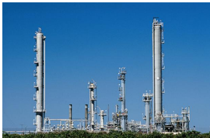
Fig.1 Industrial Steel Stacks
